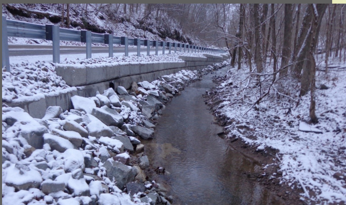
Photo: 2019 landslide repair on Cherry Road, Hopewell Township.
