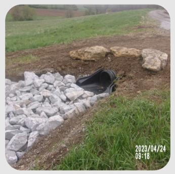
Short Cut Road Drainage project, April 2023. Poor road drainage along the roadway caused yearly maintenance required to keep the to road open during the wet season. Pictured is the outlet of one of the 9 new cross pipes being installed along with 10 ditch outlets to manage stormwater more efficiently.
