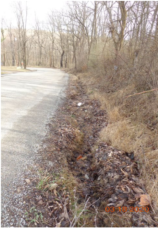
Cokeburg Hill Before: Large quantities of water run alongside the roadway in ditch causing erosion and sediment to be discharged into Pigeon Creek.
