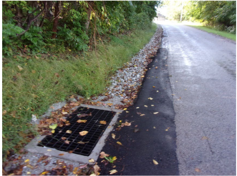
Cokeburg Hill After: Under drains and inlets were to reduce the volume of stormwater that can cause erosion in the ditch. Riprap was also added to reduce the velocity of the water and prevent future erosion. This system performed flawlessly and managed the 5 inches of rain we received on from Hurricane Ida in September of 2021.
